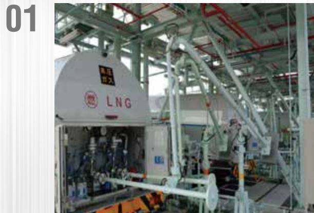
Loading Arm for tank lorry
