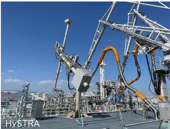
Loading arm for liquefied hydrogen in tubular steel being connected to a tanker.
