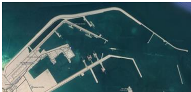
Ras Laffan LNG export port where our LA is delivered
