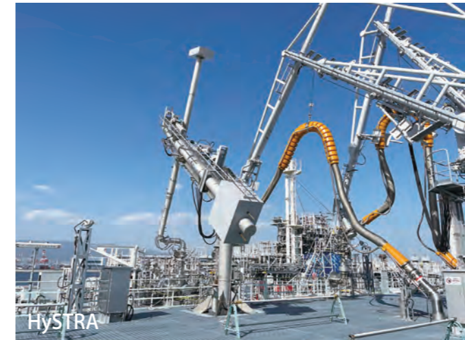
Loading/Unloading operation of 6" LH2 Marine Loading Arm
